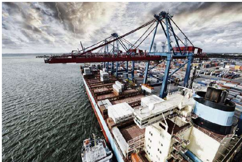
container port seen from the air
